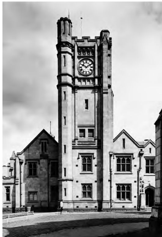
Clocktower of the Arts and Education Block (1919–24), now known as Old Arts. The building is clad in Kyneton freestone that was quarried at Lauriston on the land of the Taungurung people.
