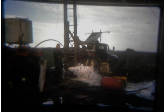
Drilling rig. ( [REDACTED] collection 1970's)
